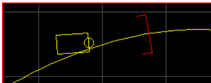
Navigation display on rig computer. Shows actual position at tunnel face
